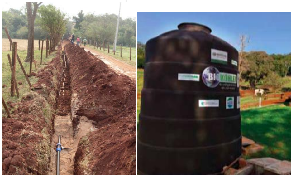
Fig. 4. Biogas collection network construction and small flow biodigestors implementation
